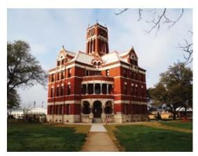
ee County Courthouse, located in Giddings, TX, was designed in the Romanesque Revival style and constructed in 1899. It was officially adopted as a Recorded Texas Historic Landmark in 1968. The Courthouse is constructed of load-bearing masonry with reinforced concrete floor slabs and steel attic and roof framing.
