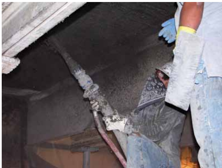
Fig. 2: Application of spray-applied mortar on double-tee flange soffit
