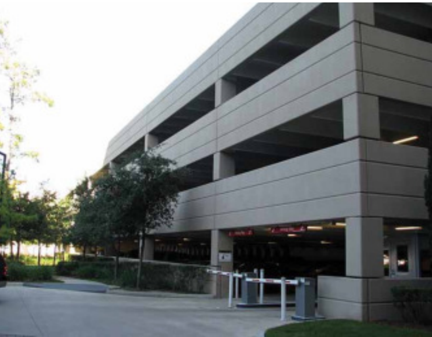
Fig. 5: Woodlands Waterway Marriot Parking Garage
