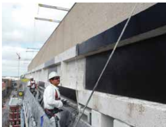
Fig. 5: Swing stage equipment used for CFRP repairs
